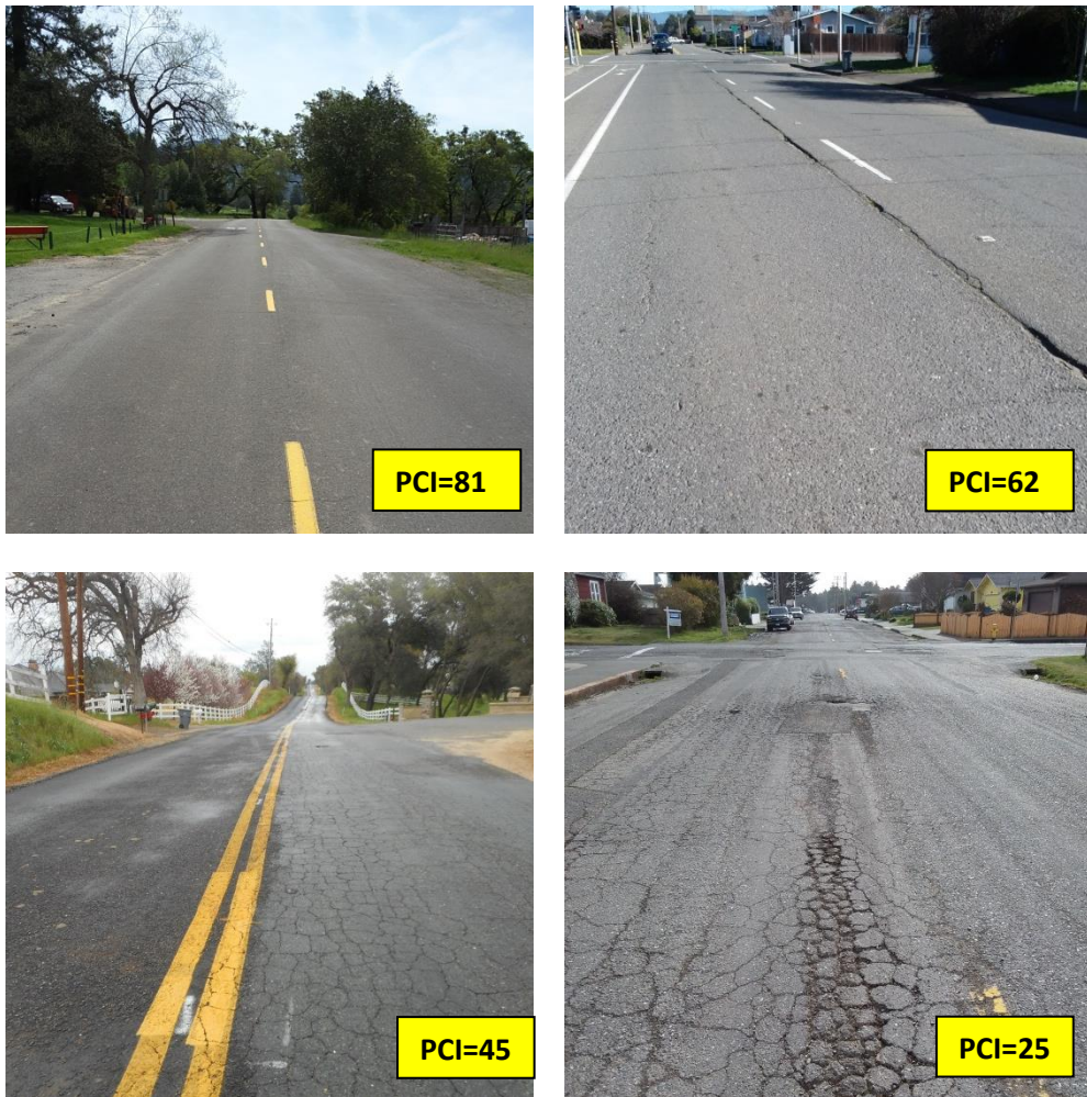
Figure 2: Examples of Roads with Different PCIs
