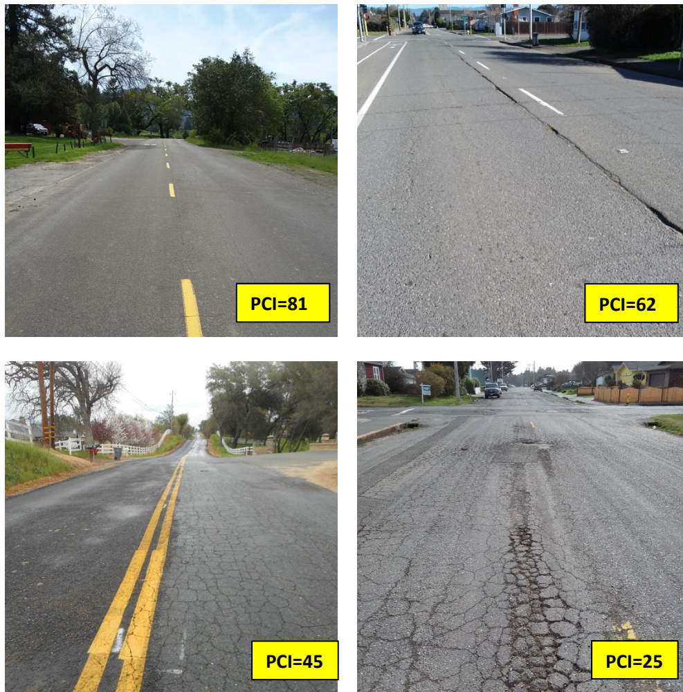
Figure 2: Examples of Streets with Different PCIs
