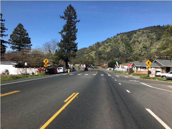
Plate 1 SR 20 at Keeling Avenue, Nice
