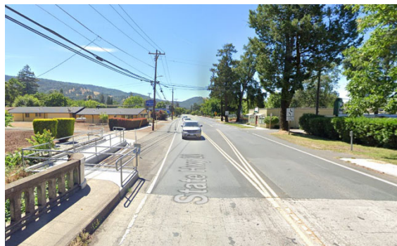
Plate 11 Two Way Left-turn Lane
