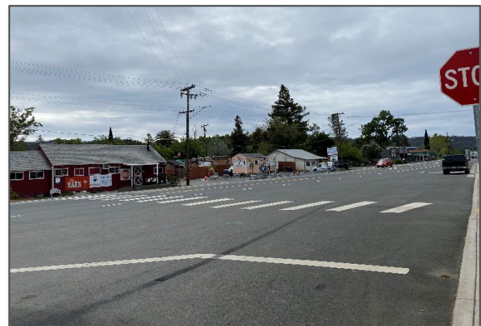
Exhibit 12. Pedestrian crosswalk near Acorn Street
