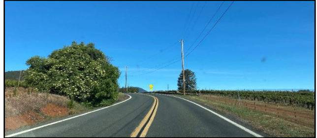
Point Lakeview Road near SR 29
