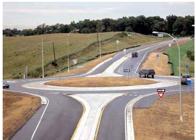
State Hwy 13 @ County Road 2 in Scott County, MN
