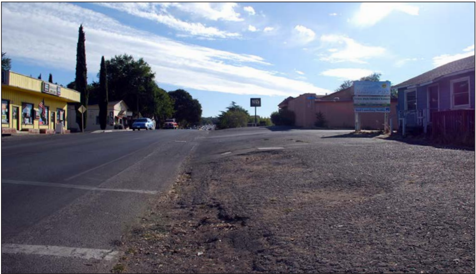
Deteriorated pavement where the roadway shoulder meets underutilized private land.
