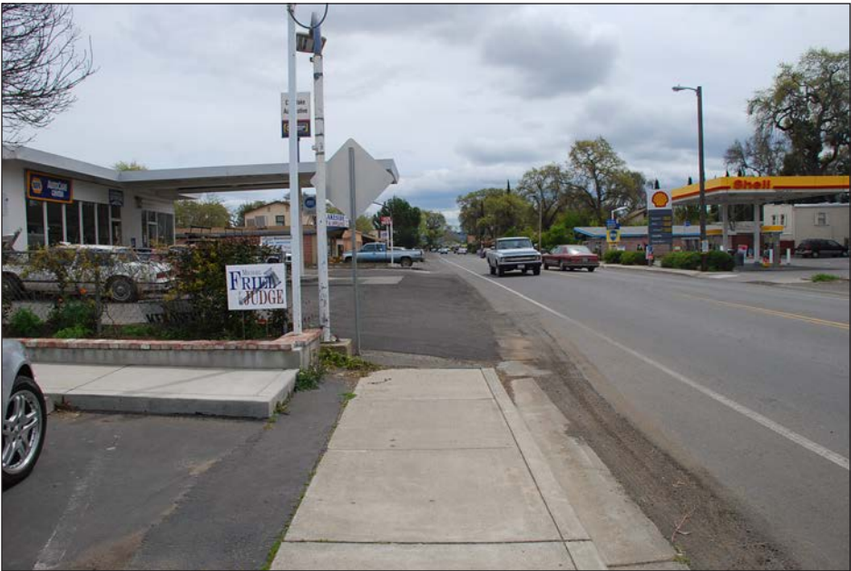
The public and private sidewalks fail to connect in the photo above. The public sidewalk ends and gives way to unlimited driveway access with no defined space for pedestrians.
