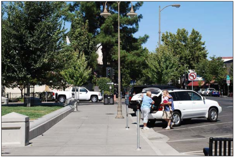
The photo shows how back-in angled parking directs passengers that are unloading toward the safety of the sidewalk.
