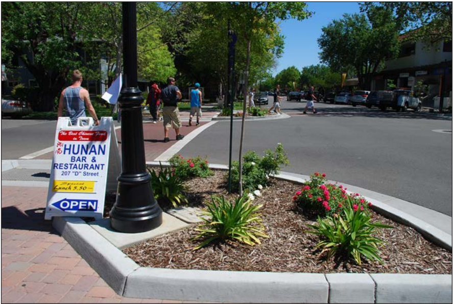
Curb extensions encourage slow vehicle turning movements, shorten pedestrian crossing distances, improve visibility between pedestrians and motorists, provide protection for cars parked on the street, and can provide added space for lighting, landscaping, signage and furnishings.
