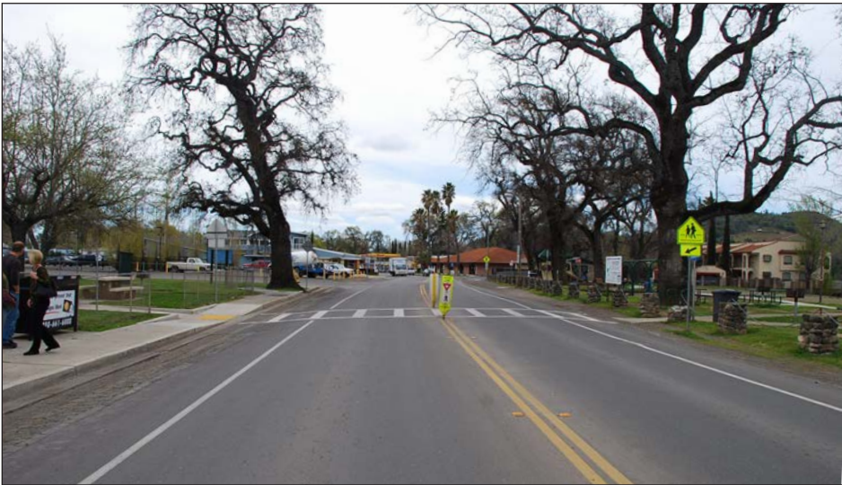
A high visibility crosswalk with lateral striping and signage is shown above on Lakeshore Drive at Austin Park. These crosswalks are more visible to motorists than two parallel lines. Added pedestrians signs also clarify to motorists precisely where to expect pedestrians and courage them to yield. Enhanced crosswalks at other locations on Lakeshore Drive would help pedestrians safely cross the street.
