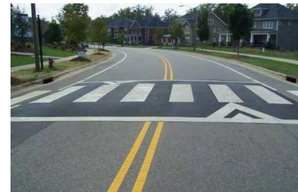
Raised Crosswalk Cruce Peatonal Elevado
