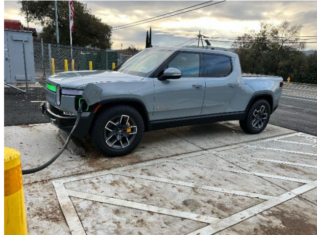
Figure 4. Clearlake Oaks charging station.
